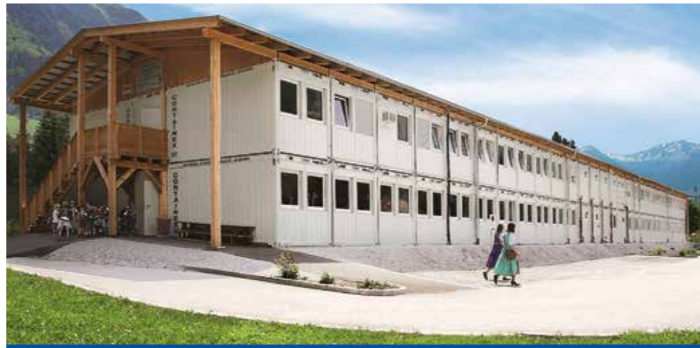
Two storey school with secondary roof
