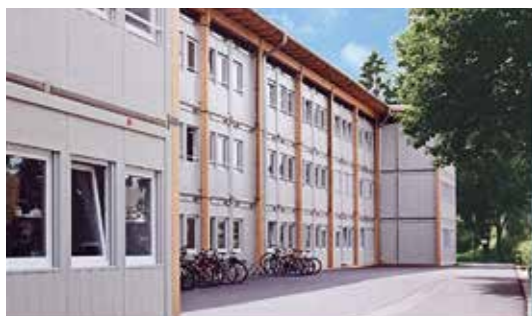
Three storey school with secondary roof
